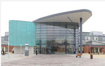
The new £400m City Hospital
